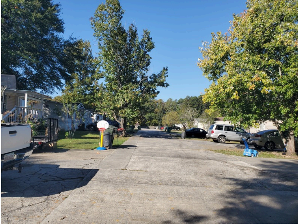
13. Typical view of the asphalt drive way
