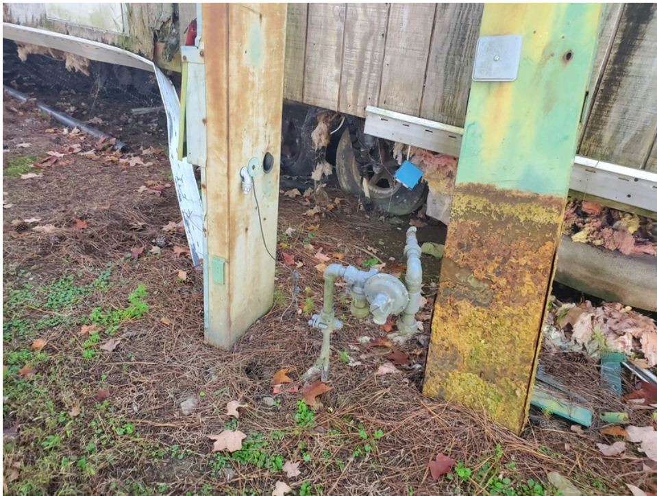
10. Natural gas hookup for a manufactured home
