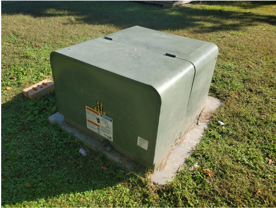
9. Typical pad-mounted transformer
