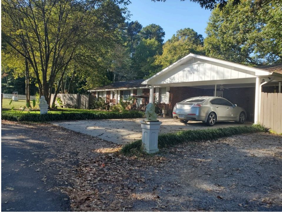
23. West adjoining residence
