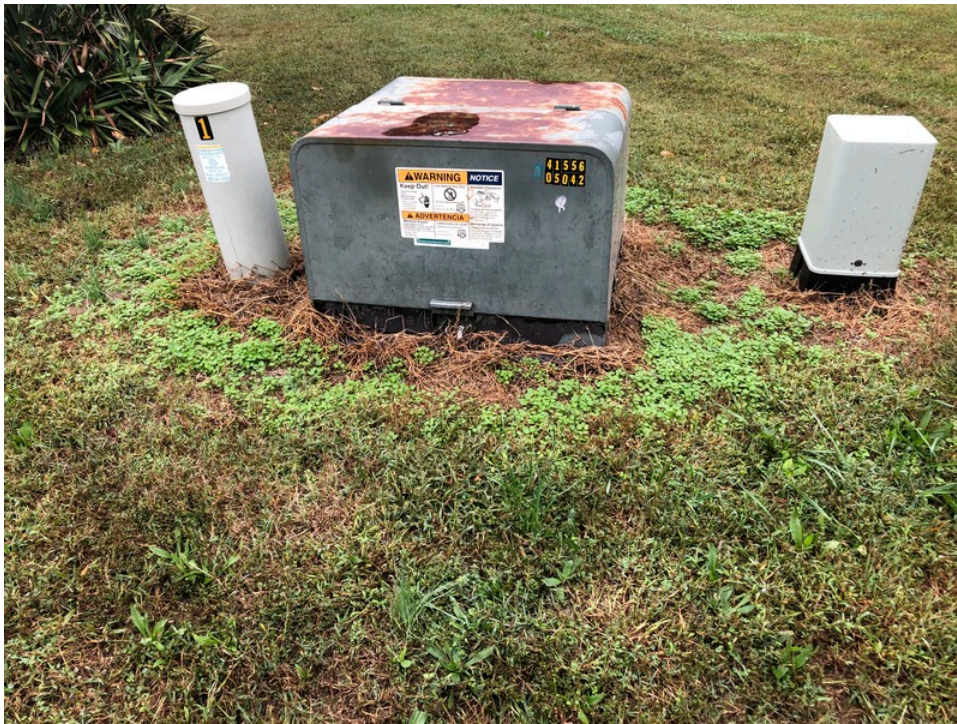
10. Pad-mounted transformer-typical
