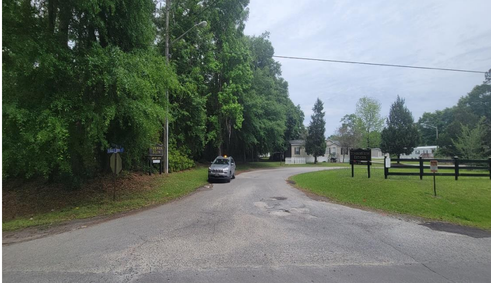
Figure 1. Main Entrance, Troupeville Road
