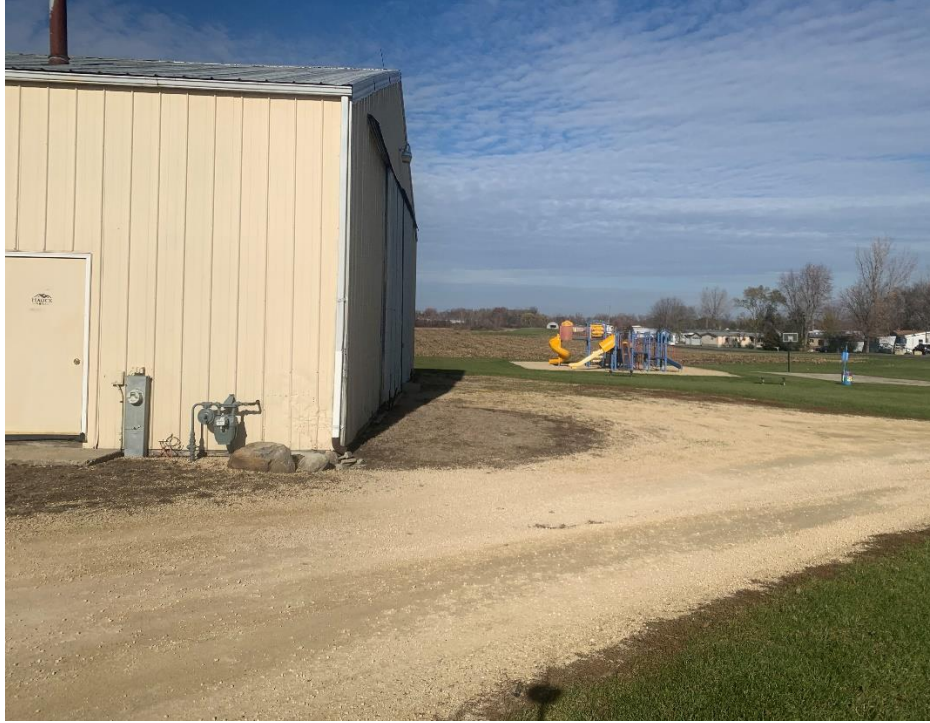
Figure 3. General Picture at maintenance building
