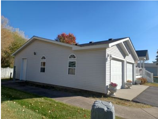
7. exterior of central storm shelter/garage
