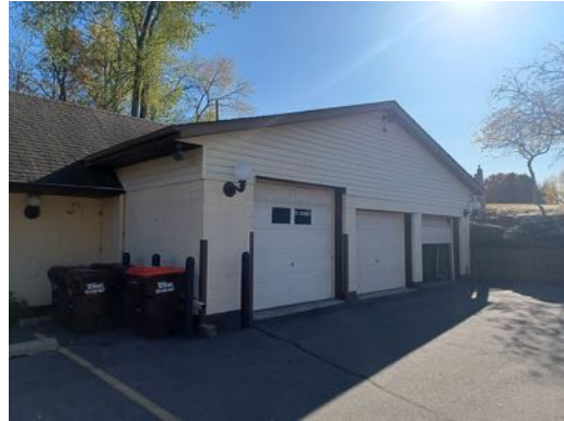
2. maintenance garage attached to leasing office structure
