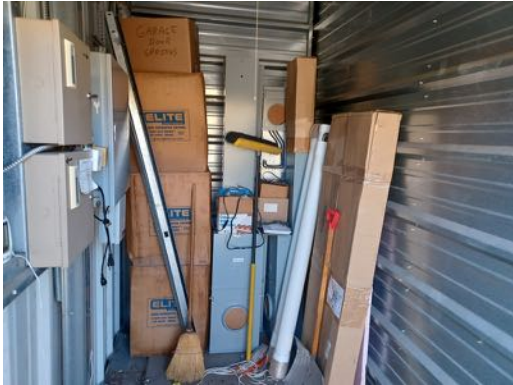
30. typical storage garage interior
