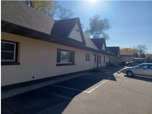
1. northern side of the leasing office structure
