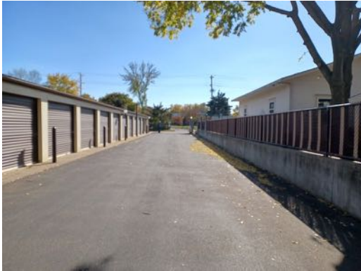
10. storage garage drive area
