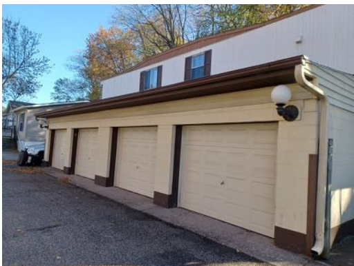
5. Property owned garage structure
