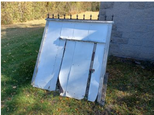
17. Housing for irrigation well
