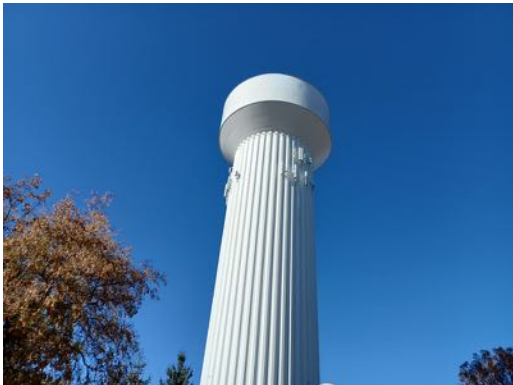
33. northern adjacent water tower
