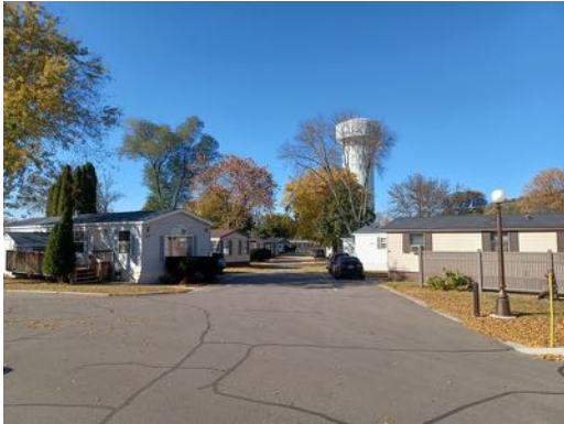
13. center of Phase I of the MHP looking north
