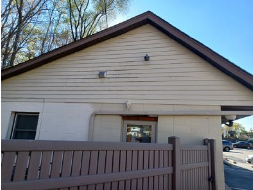
3. eastern side of the leasing office structure
