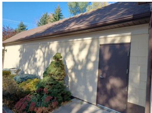
6. storm shelter exterior
