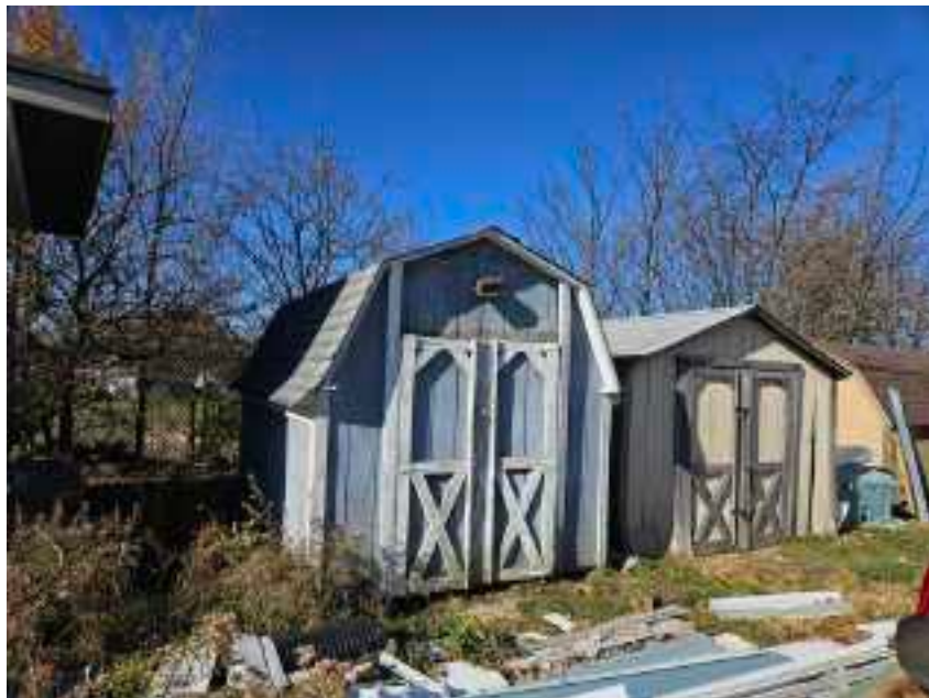
20. Maintenance storage barns
