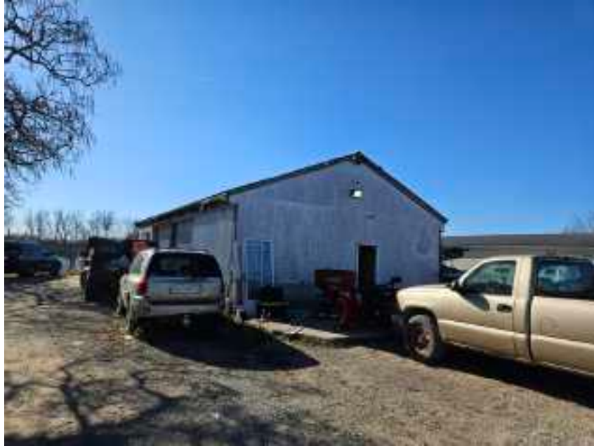
17. Maintenance barn exterior
