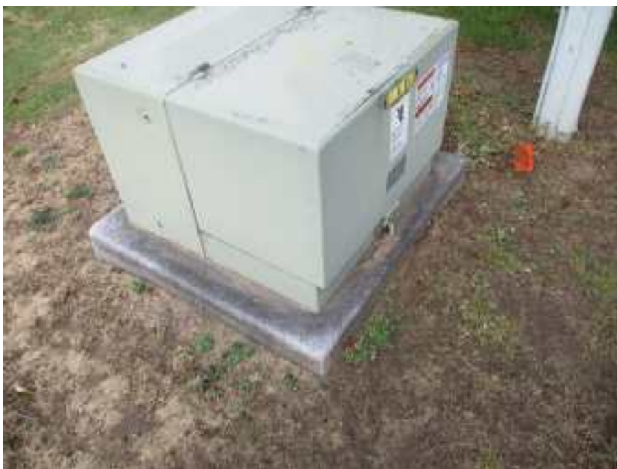
Typical pad mounted transformer
